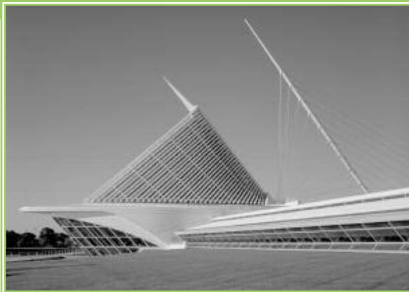
Milwaukee Art Museum (WI): Bridge to museum (wings are opened and extended when wind speeds are safe). Saarinen, Kahler, Calatrava.
