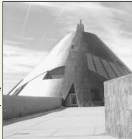
University of Wyoming Art Museum: East end of museum from upper level, showing outdoor sculpture court. Predock.
